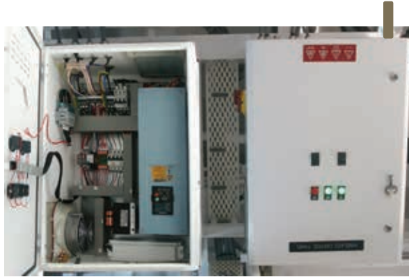
Windlass control panels with frequency converters
